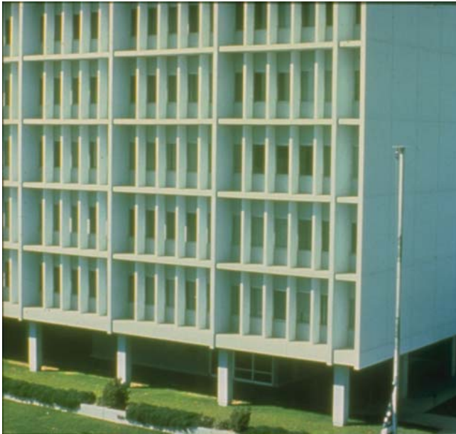
(a) A view of the building
